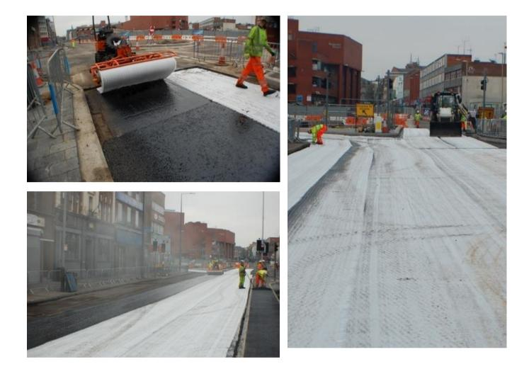
**TOP LEFT:** Asphalt Grid Systems bespoke laying machine, incorporating a hydraulic pretension mechanism to apply an even tension when installing.
